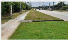
• Upgraded the drainage channels along the buffer zone connected to public roads to prevent hazards caused by soil erosion onto the road surface and to mitigate road damage from external water runoff eroding the buffer zone.
